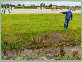
Drains throughout the site protect the ground from flooding and feed the arena surfaces
